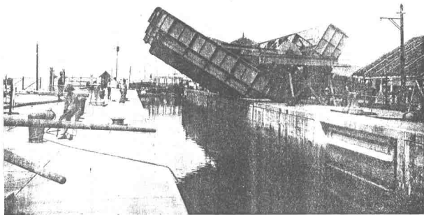
JOHORE CAUSEWAY. ROLLING BRIDGE CARRYING ROAD AND RAILWAY TRACKS ACROSS LOCK.
